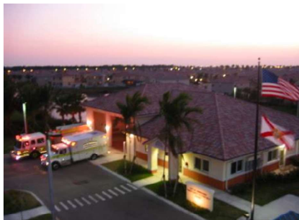
Greenacres Public Safety Station No. 2 - 2002
